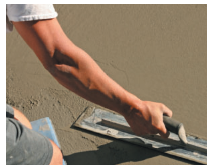
Float finishing a cement sand screed
