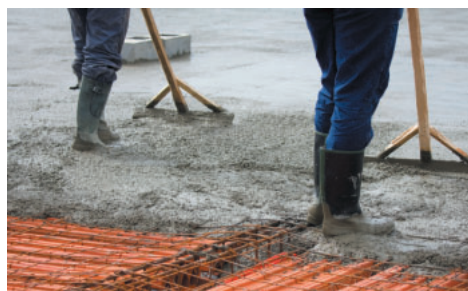
Placing an in-situ reinforced concrete floor
